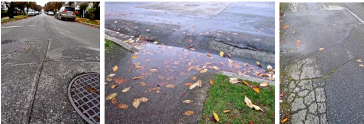
The state of the asphalt along a stretch of the site of act 2, “The Swamp.” Notice the buckles, bends, and cracks in the pavement as of November 2012. Photographs by author.
